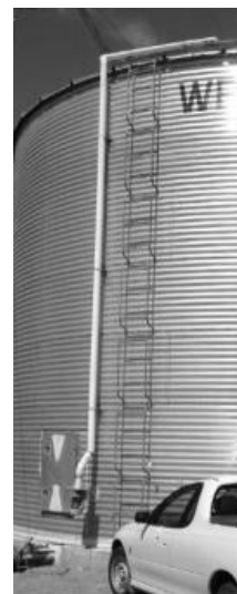
Fig. 1 Recirculation system fitted to 835m silo
